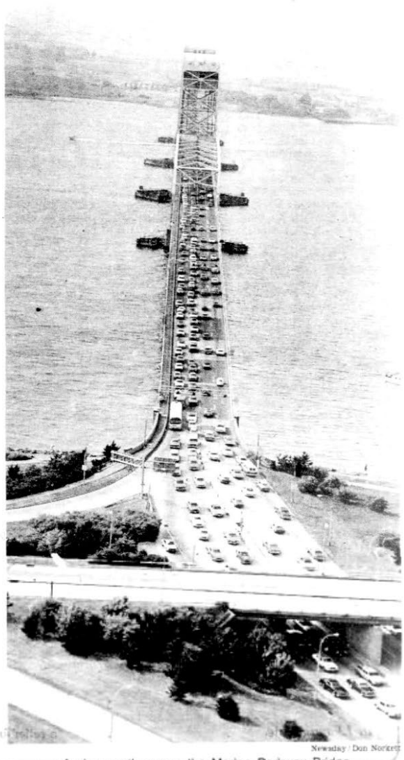
A view north across the Marine Parkway Bridge
