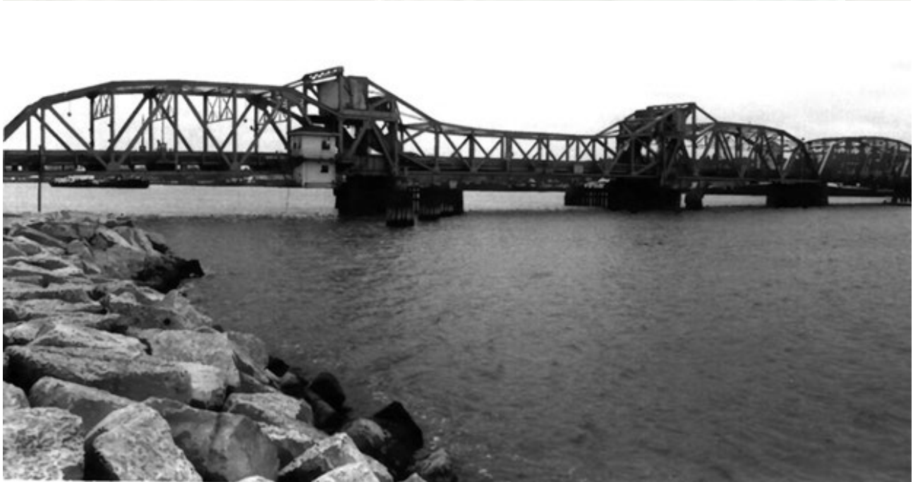
The Sturgeon Bay replacement Bridge is the only overhead truss, Scherzer-type, double-leaf, rolling-lift Bascule Bridge that remains in Wisconsin. Completed in 1931 the center section splits and lifts \frac{1}{2} to each side to allow large boat passage.
